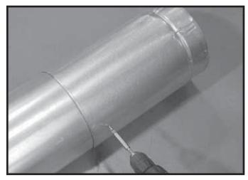
Figure 10.7 Screws into Slip Section
